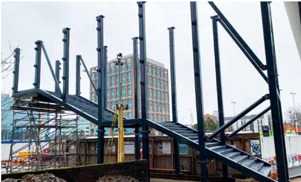
Coventry Station Design, surveying, modelling and fabrication and delivery of structural steelwork for the new Coventry Station
